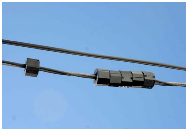
Fig 31 – Chokes on a Power Line (the bare conductor is the neutral, and is grounded)
